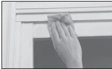
1. Use mild soap and water or alcohol to clean the surface of the door frame. (The door frame must be completely dry before mounting the Sliding Door Genie™).
